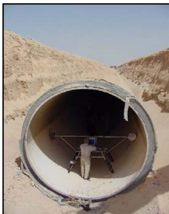
Figure 15 -- Electromagnetic Inspection and Acoustic Monitoring using Hydrophones
