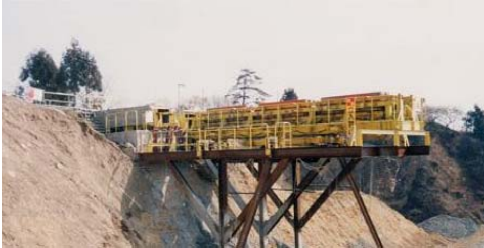
Figure 4 Capsules reaching the end of the Akima PCP to discharge their load at the dump site (Courtesy of the Sumitomo Metal Industries, Ltd.)
