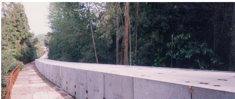
(b) PCP extending outside the tunnel to the dump site
