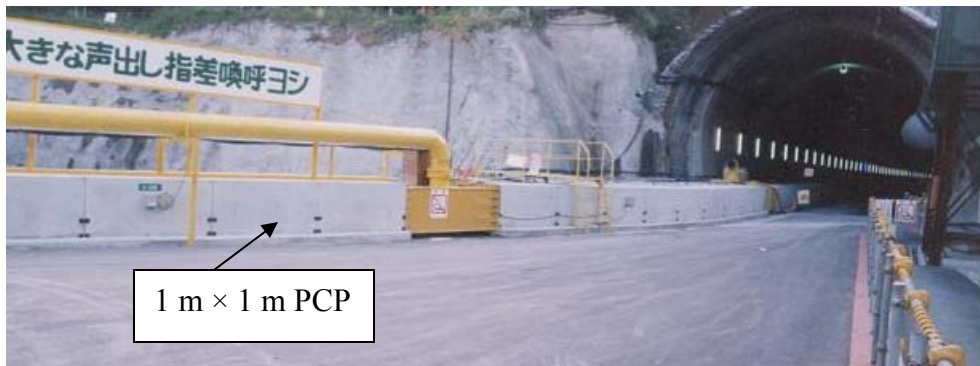
(a) Tunnel entrance
