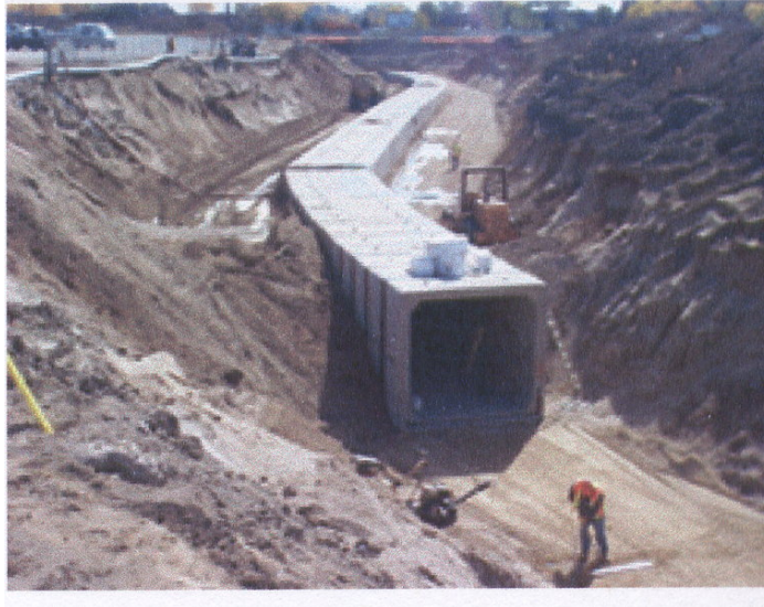
Figure 25 Large box culvert made of reinforced concrete that can be used for constructing large rectangular conduits for PCP using the open-cut construction method. (Photo reprinted from the web page of the Hanson Pipe & Products, Inc. [45])
