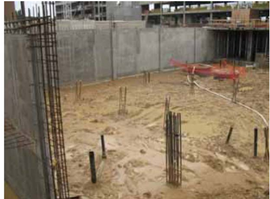
Area C – First floor deck rebar and basement sub-grade
