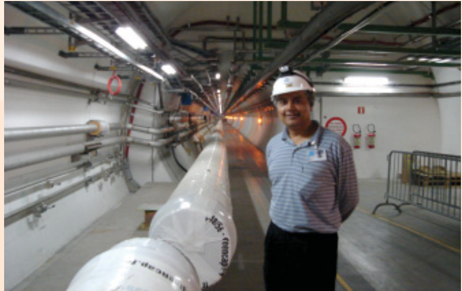
Physics professor Kaushik De, Director of the Southwest Tier 2 Center, in the LHC tunnel in Geneva, Switzerland. The LHC tunnel forms a circle 27 kilometers long, 100 meters under the surface, straddling the countries of France and Switzerland.
