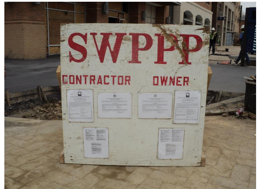
Large Construction Site
